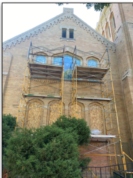
Stained glass work, West Façade
